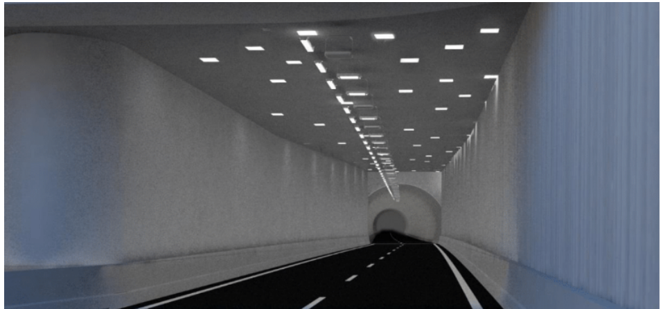
Parans Solar Lighting for a tunnel entrance zone. (Source: COMOL5)
