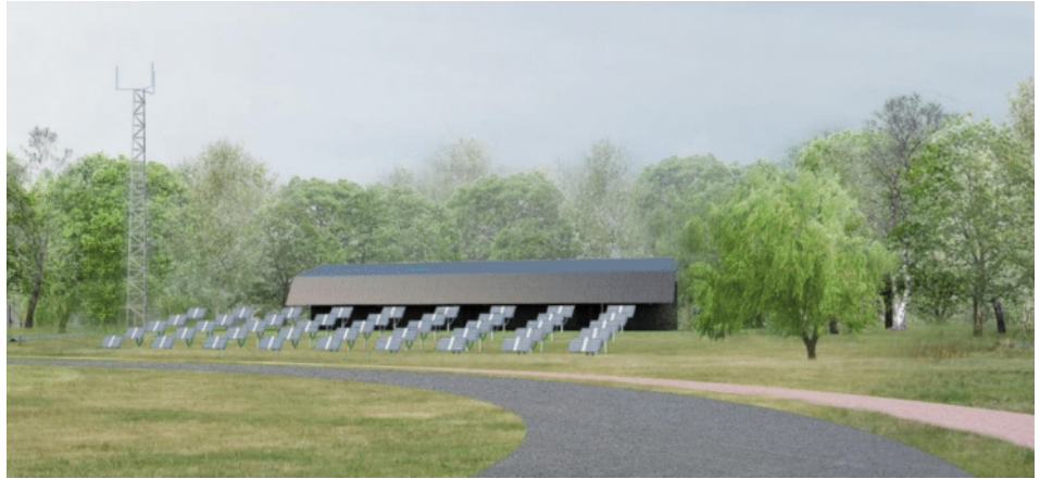
Parans sun collector cluster situated above the tunnel. (Source: COMOL5)
